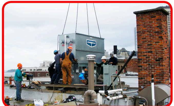
Cooling Tower Replacement Grand Central Building - Seattle, WA
